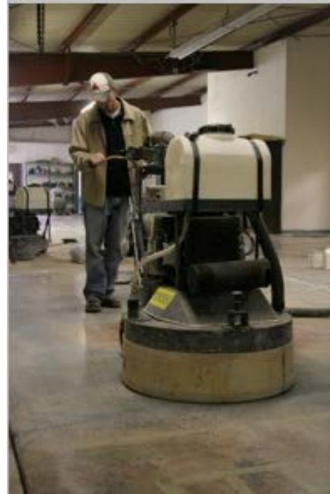
Figure 2: Floor polishing tool with water control (Courtesy of the Concrete Polishing Association)
